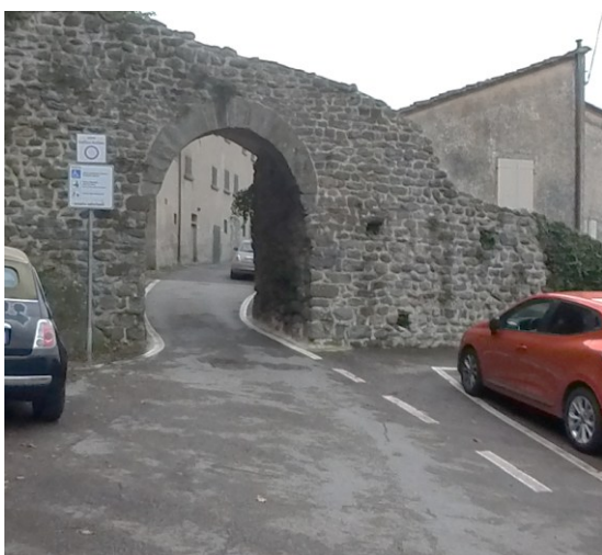
2 Gate of Via Larciano
