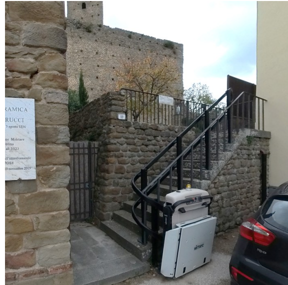
9 Stairlifts for access Rocca
